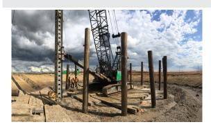
anchors were centered into each pile, drilled into the bedrock, and grouted in place to provide a stronger outcome than what was originally required.
