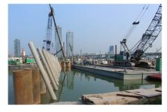
that had frequent boat traffic. To overcome this challenge, SB Canada developed an installation template that utilized previously installed pipe piles, temporary spuds, and GPS survey equipment to ensure proper location. The template was independent of the barge and was therefore not impacted by waves and/or barge movement
