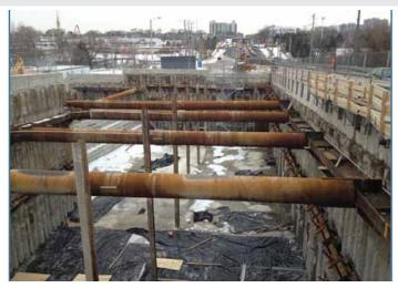
A total of 305 caissons were drilled, ranging in size from 880 to 1300mm in diameter. These caissons were some of the deepest SB Canada had to date. With a range in depth from 20 to 36m, a total of 3 rigs ran simultaneously, 24 hours a day, during optimal production. With focus on precision and keen attention to detail, not only was the project a sucess, but it also estiblished a first for SB Canada.
