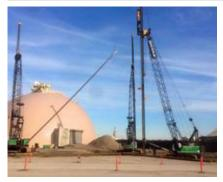
length piles, SB Canada reduced the total pile installation by a month. See the photo above of Berminghammer VTL System lofting a 100 foot pile.
