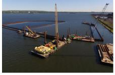
footwork with its falsework. "We can't put in excessive amounts of falsework because that would disturb the lakebed material. So, we actually implemented a floating template system," Jeff Thomson explained. "We mounted our falsework onto a smaller sectional barge and held that in place with temporary spuds. We can move it along the length of the wall as we install it. That limits the amount of disturbance."
