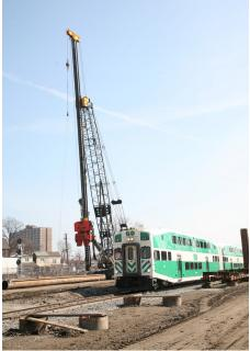
production method one could imagine. The installation of the final piles finished in late summer of 2010, just in time for us to be awarded the contract for the second phase - drill out and concreting of the driven pipe piles.
