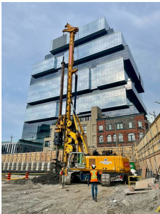
Proximity of a high-rise building to the drilling area.
