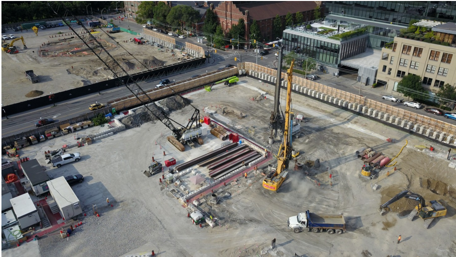
Aerial photo of the north shaft of the station
