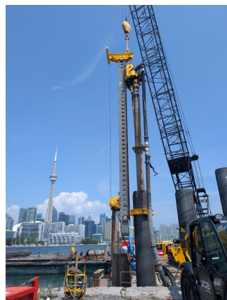
Hanging Lead System to install the pipe piles for the combi-wall
