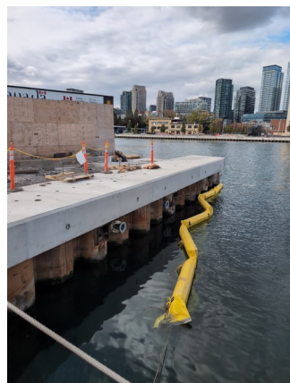
Completed dock wall with precast concrete coping
